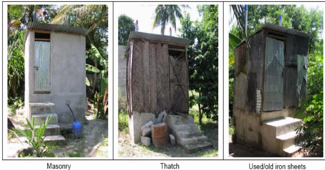
Figure 2. Examples of EcoSan dehydration toilets with urine-diversion in Tanzania using Local Material [13]
