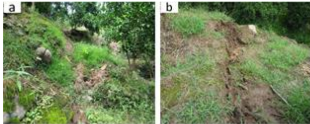
Figure3. Photographs of the Ground Cracks in the Middle Part of the Eastern Landslide in July 2007
