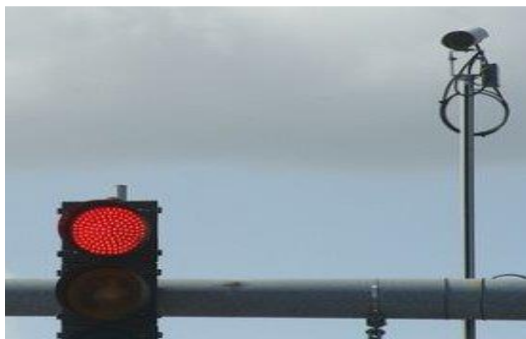
Figure 1. Automatic Camera over Intersection to Catch Red-Light Runners
