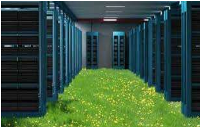
Figure 6. Green Data Center
