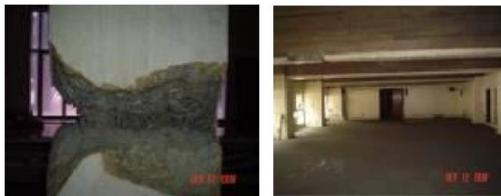
Figure 4. Typical level tested by GHD and inside the GSIS building
