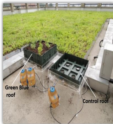
Figure 4. Green Blue Roof Cheong-un Middle School
