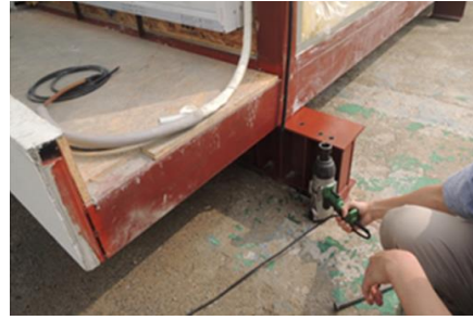
(b) Work that prohibits the use of electric impact wrench
