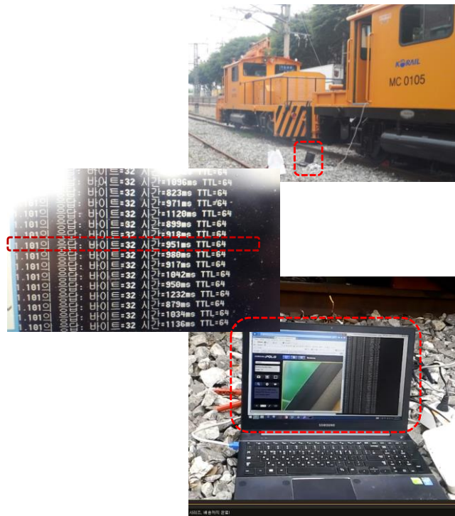
Figure 6. Photos of Rail Track PLC Test between EL and Rail Track
