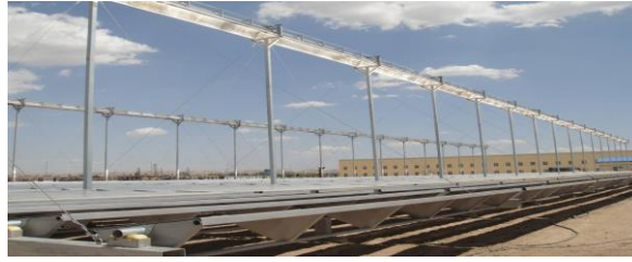
Figure 2. Tracking Picture of Linear Fresnel Collector
