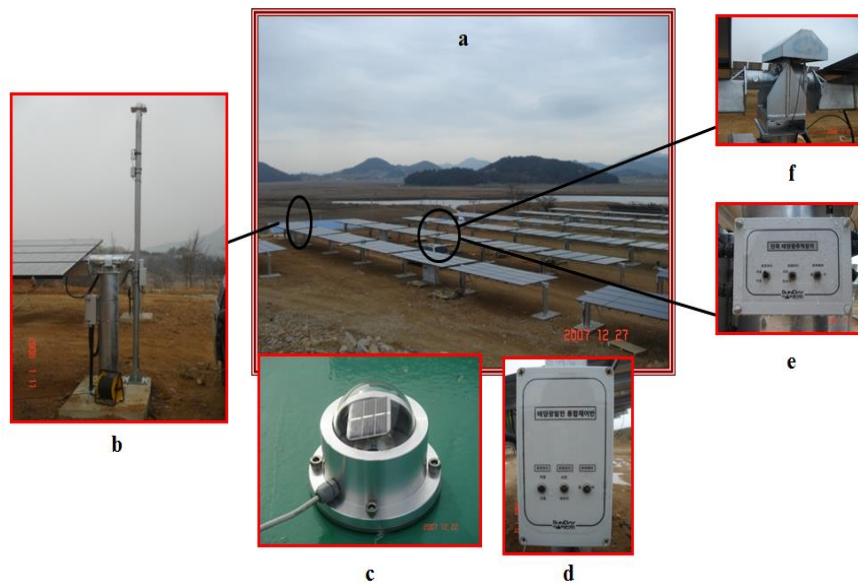
Figure 2. The 1 Axis Solar Tracking Unit (A) 6 Section Reduce Solar Tracking Device, (B) Integrated Remote Control Panel, (C) Ambient Light Sensor, (D) Integrated Control Panel, (E) Board, (F) Speed Driving Unit
