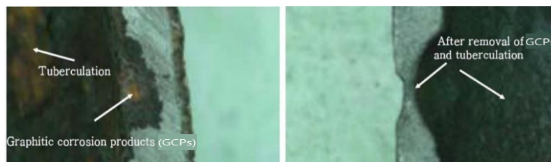
Figure 1. Pictures of CIPs before and after Shot-Blasting
