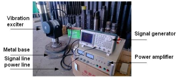
Figure 6. Exciter and Signal Transmitting Devices
