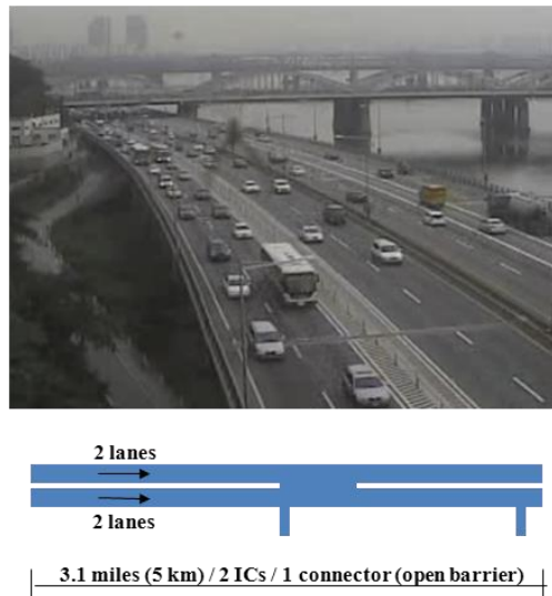
Figure 1. 88 Olympic Expressway in Seoul, Korea ( www.smartway.seoul.kr )
