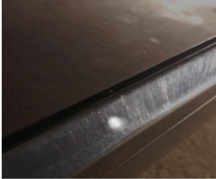
Figure 5. Dirt on the Tracks
