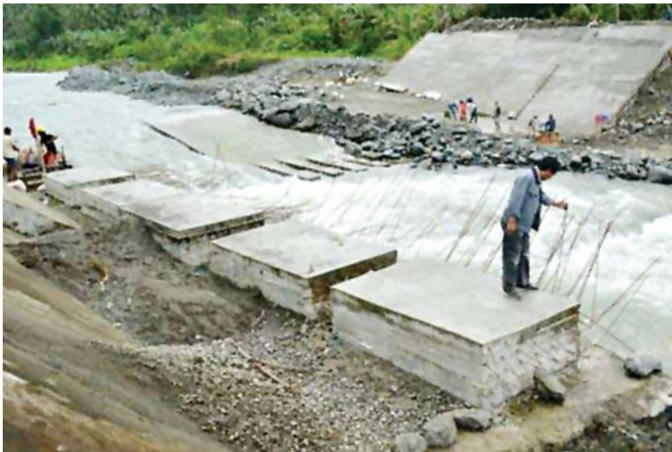
Figure 4. Ground Works of the 17M php Dam of Communal Irrigation System
