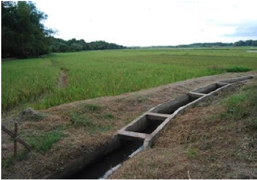
Figure 1. Infrastructure Project to Irrigate 124 Hectares of Land
