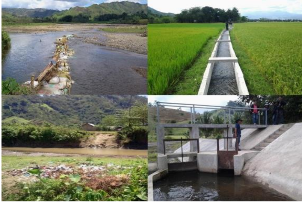
Figure 3. Communal Irrigation Project
