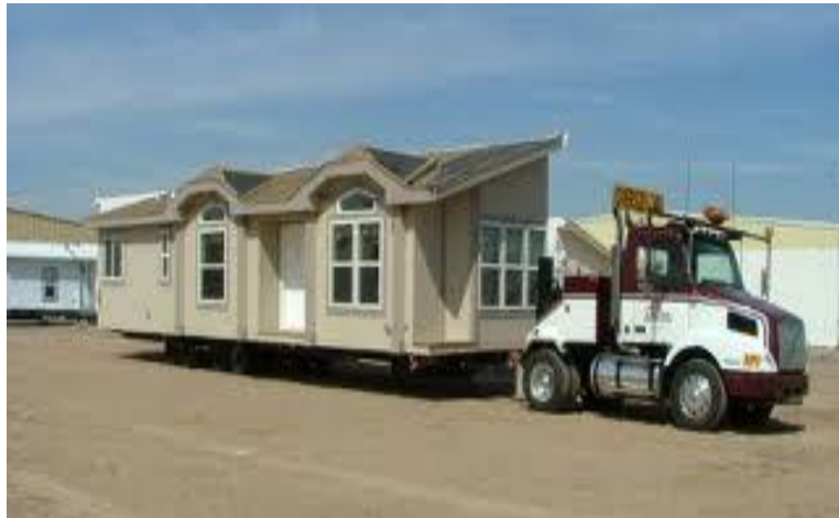
Figure 4. Transporting of Modular House
