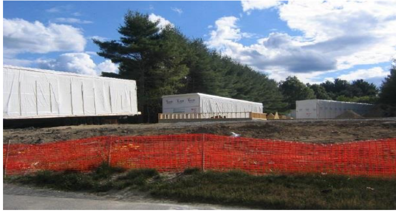
Figure 22. Modules are Stuck by Crane
