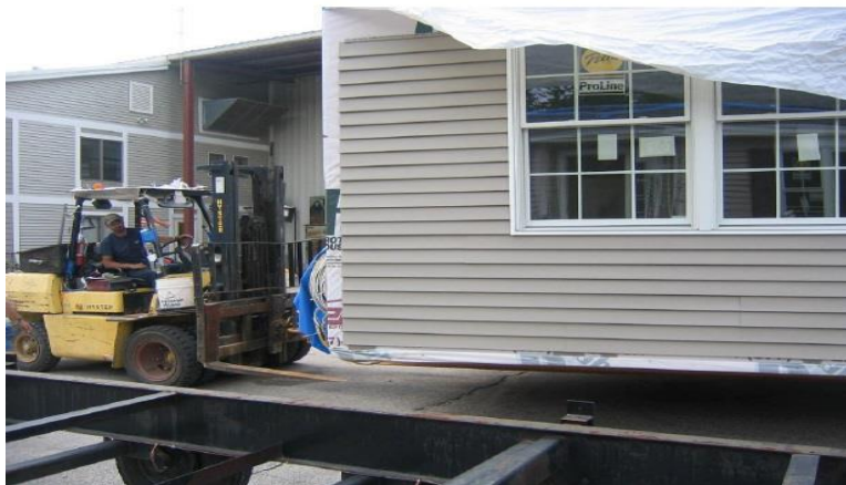
Figure 17. Transporting of Modules
