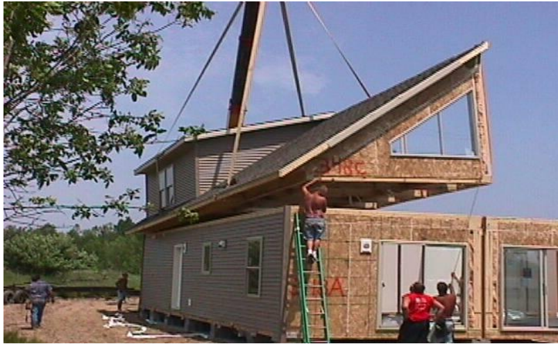
Figure 11. Modular House Assembling
