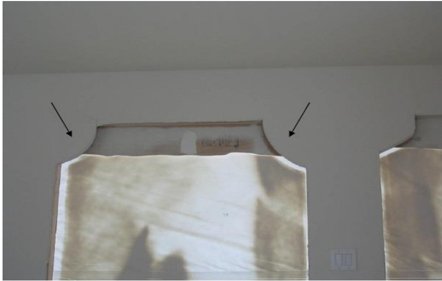
Figure 18. Sheetrock is Cut with Extra Slack
