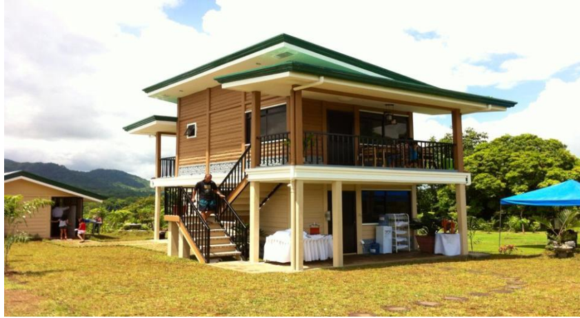
Figure 13. Modular House Assembled on Site
