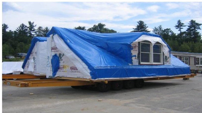
Figure 21. Modules are Carefully Secured to the Truck
