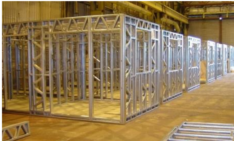
Figure 6. Steel Frame Construction
