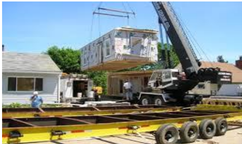
Figure 12. Modular House Delivery
