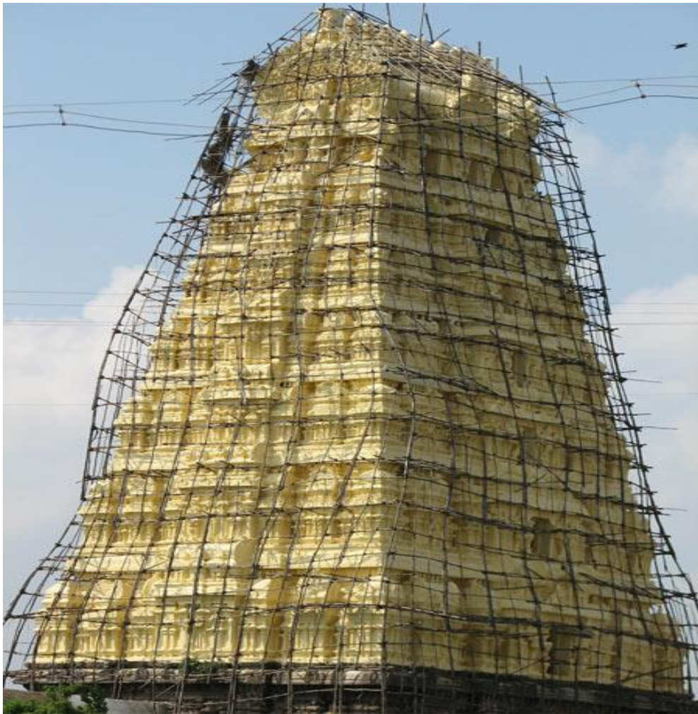
Figure 1. Bamboo used as Scaffolding
