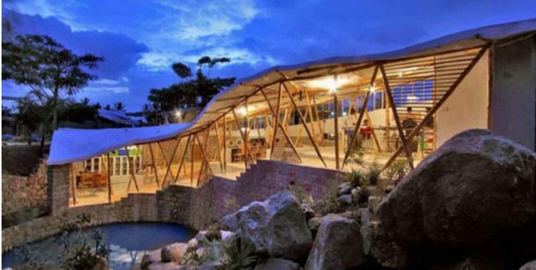
Figure 8. Bamboo Symphony Office Building
