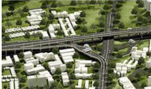
Figure 3. Main Toll Plaza section
