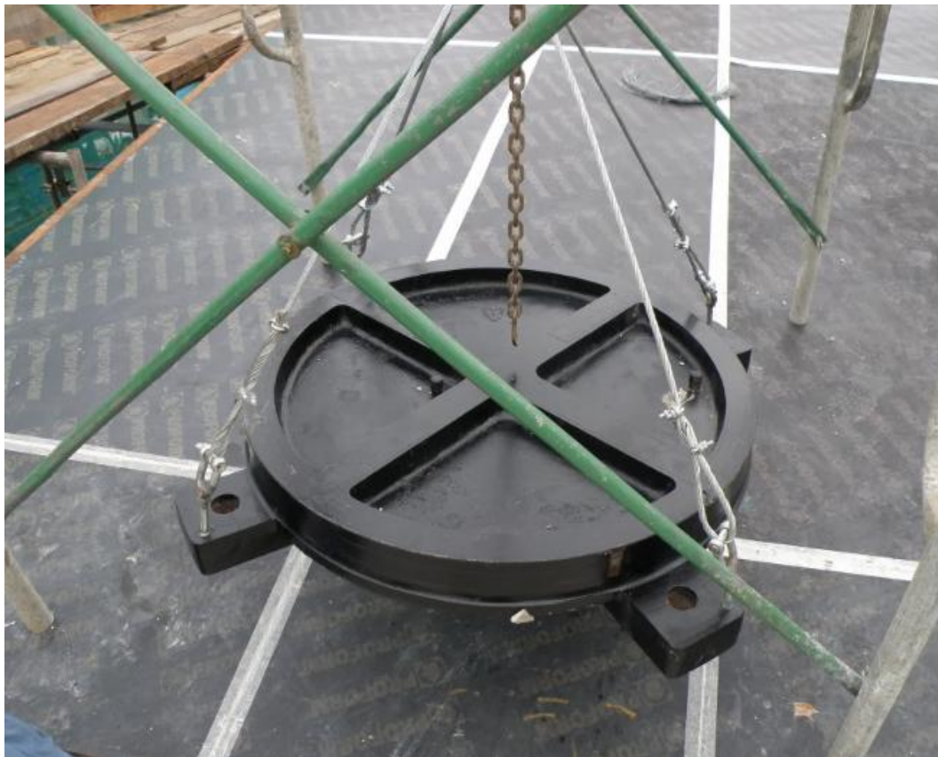
Figure 6. Sequence installation of sosrobahu mechanism
