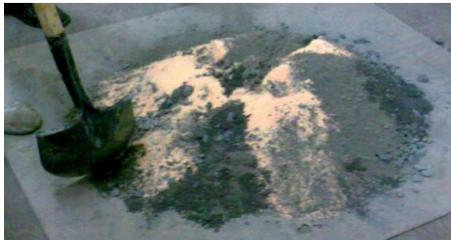
Figure 3. Mixing the thermoplastic
