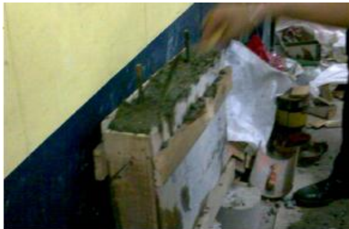
Figure 5. Pouring the mixture into the forms
